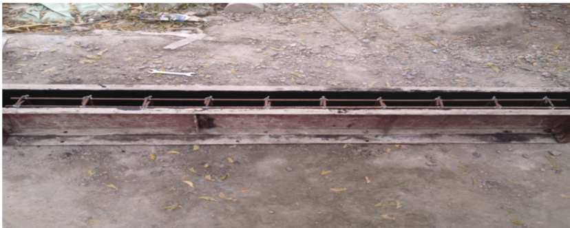
Fig 4. Beam mould with Reinforcement
